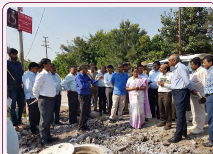
Spot Visit at the site of Sewer Death at NOIDA.
